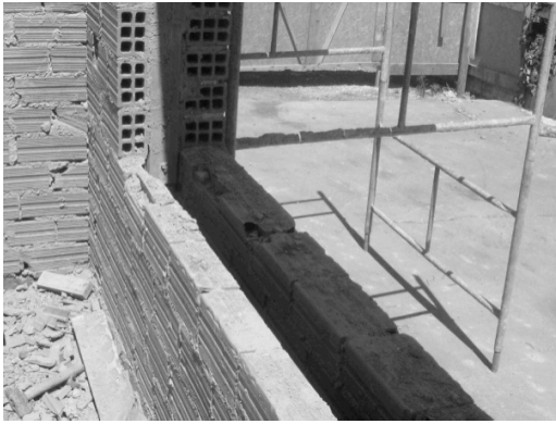
Figure 6: Double brick walls with cavity
